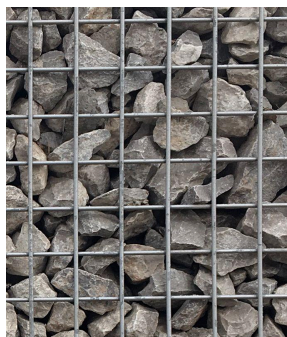
Stone-filled mesh screen
